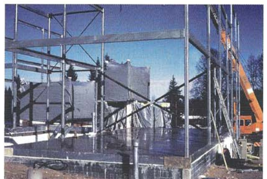
Fig. 21 Combined system in light-weight steel construction A load-bearing wall structure is added to the steel skeleton (Rautaruukki Oyj, Finland)
