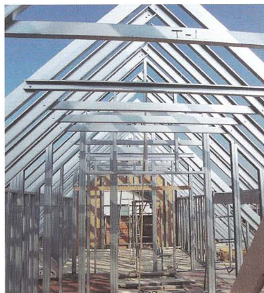
Fig. 10 Roof truss of a residential building made of cold-formed steel profiles (The Japan Iron and Steel Federation, Japan)
