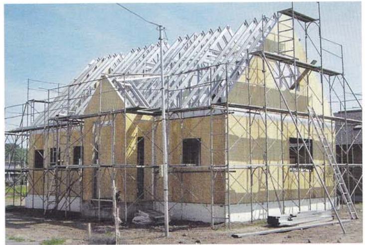
Fig. 17. Building in light-weight steel construction (The Japan Iron and Steel Federation, Japan)
